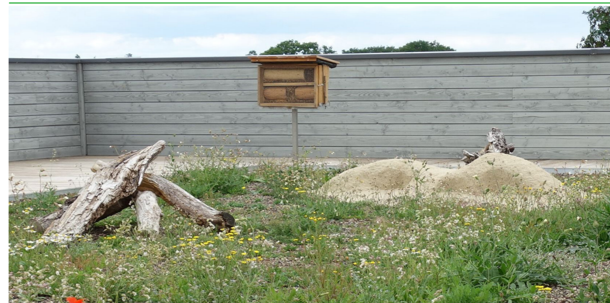
Figure 2: Nesting structures for insects on a green roof with native plants: deadwood, sand mound and high-quality nesting aid made of reed stalks and spot-drilled dead wood of deciduous trees.
